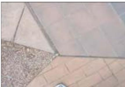
*Avoid placing multiple paving surfaces in the walkway.*
