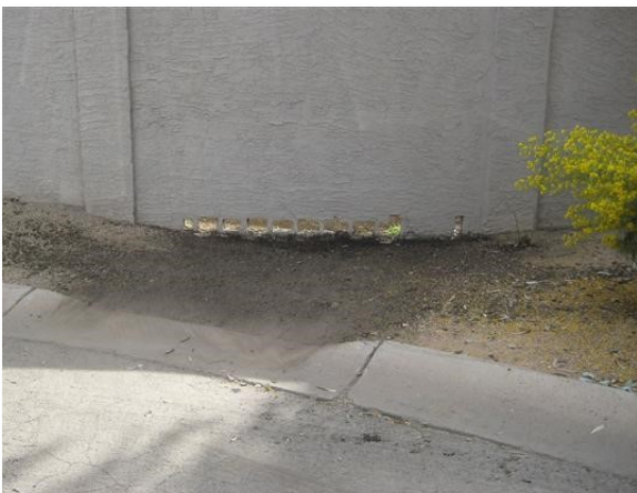
Weep holes easily become clogged, preventing water from flowing through.
