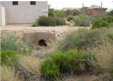
Example of a culvert designed to carry runoff.
