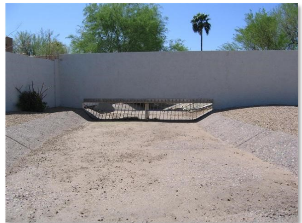
A wall with a trash rack built over a drainage easement maintains a clear, open area from which water can travel.
