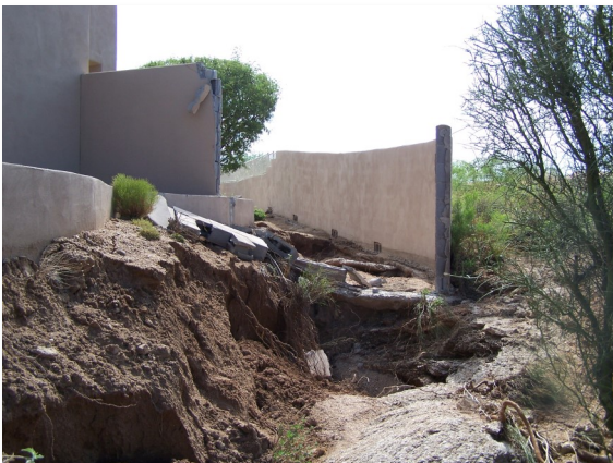
A wall located within a wash fails due to erosion.
