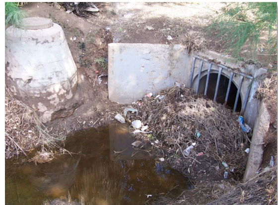
Examples of areas requiring maintenance: A wash needs to be cleared of overgrown and dead vegetation (left), a grate needs to be cleared of debris (right).
