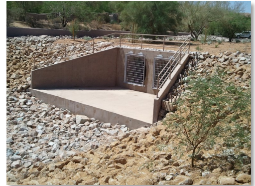
The image above shows how a piped system routes stormwater to a basin.
