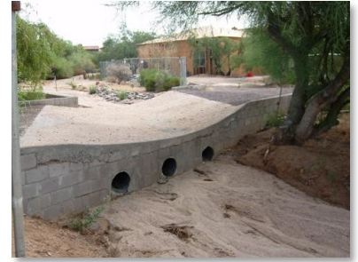
The example above shows the necessary dip and slope of a driveway with culverts built over a wash.
