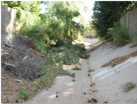
Examples of areas requiring maintenance: A wash needs to be cleared of overgrown and dead vegetation (left), a grate needs to be cleared of debris (right).
