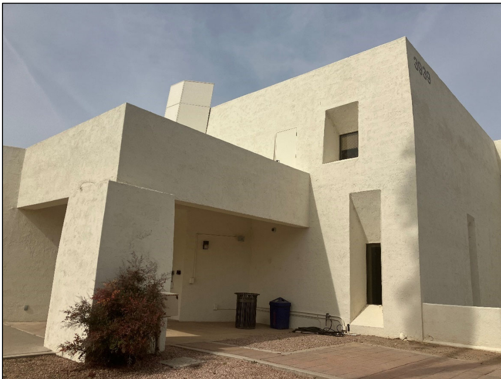
Photo 11. View of porch on the east elevation. View facing northwest (Logan Simpson, 2023)
