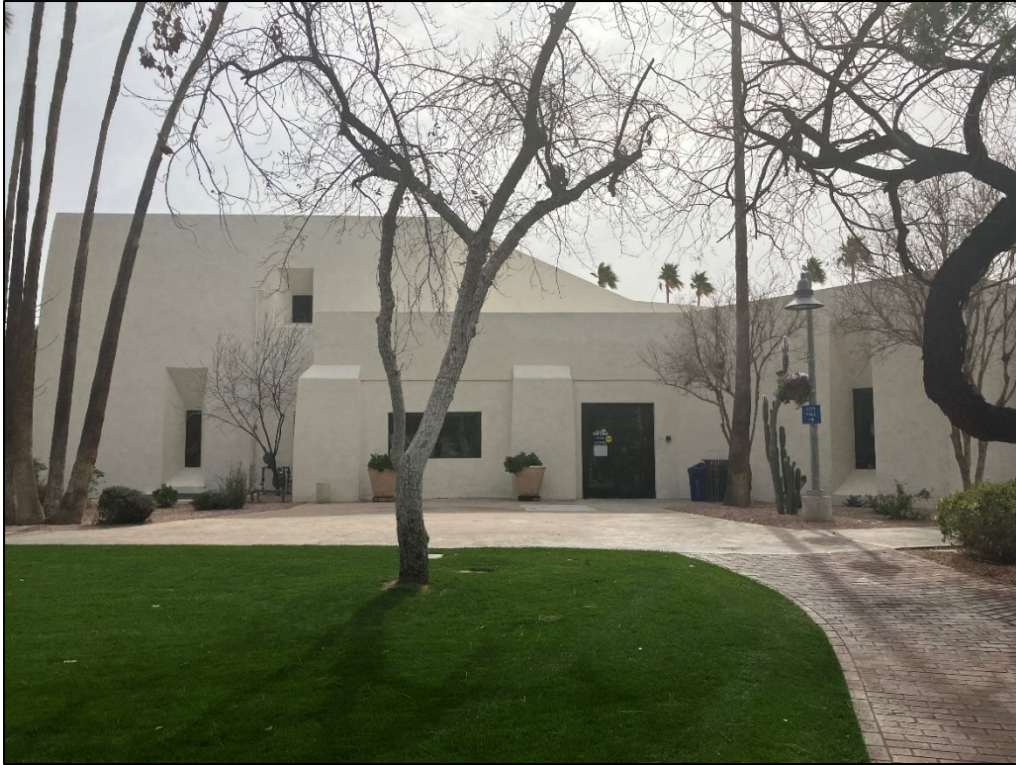
Photo 8. View of staff entrance on the north elevation. View facing west (Logan Simpson, 2023)
