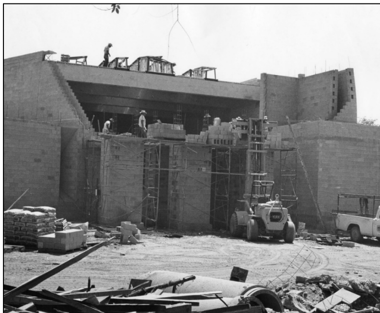
Photo 3. Historic view of the west elevation under construction. The double concrete block walls and beam construction can be clearly seen, c. 1967 (Scottsdale Public Library)
