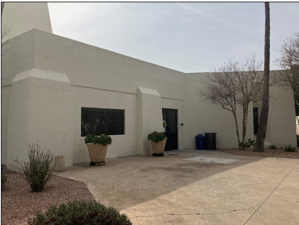
Photo 9. View of staff entrance on the north elevation. View facing northwest (Logan Simpson, 2023)
