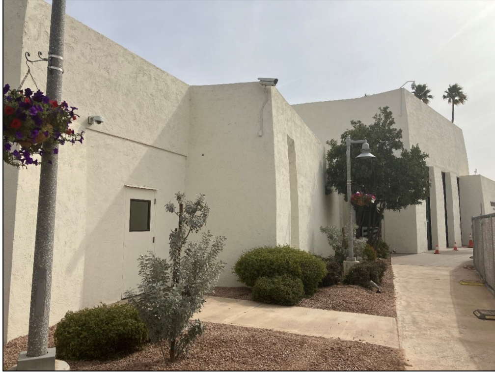
Photo 6. View of west elevation. View facing southeast (Logan Simpson, 2023)
