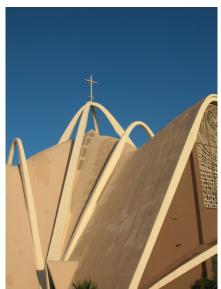
Expressionist architecture was often the result of a collaboration between an innovative architect and engineer. The same architect and engineering firms were responsible for the thin-shelled concrete Los Arcos Methodist Church south of McDowell Road.
