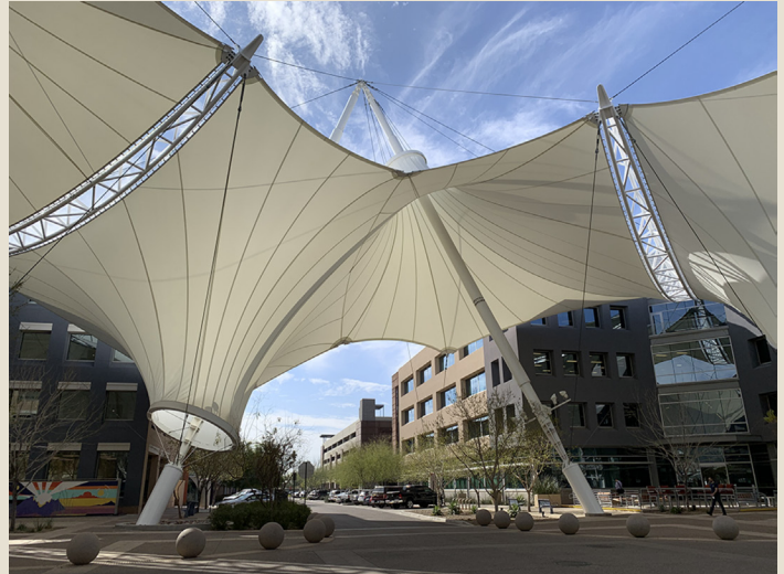
SkySong shade structures strengthen area identity while providing filtered shade.
