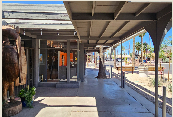
Flat roof covered walkway is constructed of wood to reinforce the pedestrian character of Old Town.
