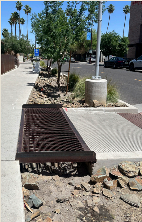
Pedestrian bridge over bioswale.
