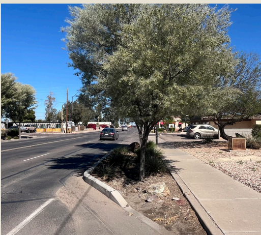
Curb extension with curb cut and bioswale.
