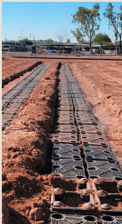
Suspended pavement soil cells.
