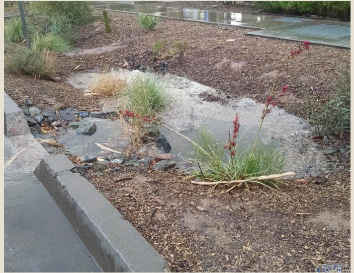
Curb cut and bioswale.
