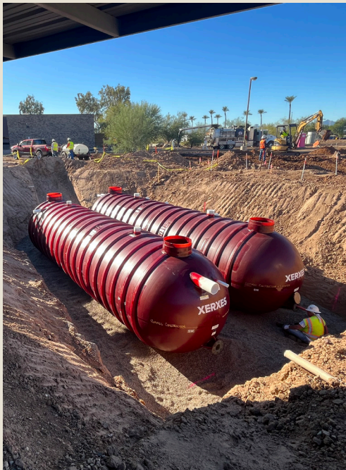
Below ground cistern.
