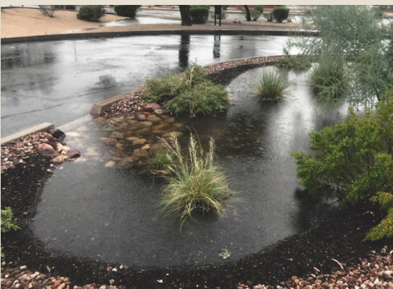
Curb cut and landscape basin.
