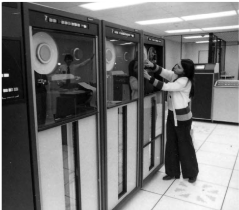
1975 Computer data center
