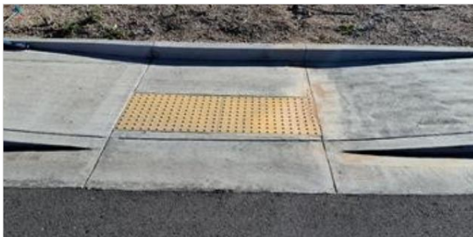
Diagonal Curb Ramp with Domed DWS
