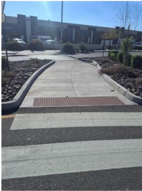
Fully Compliant Median Refuge Island
