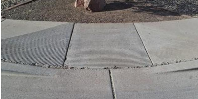
Diagonal Curb Ramp with Textured DWS
