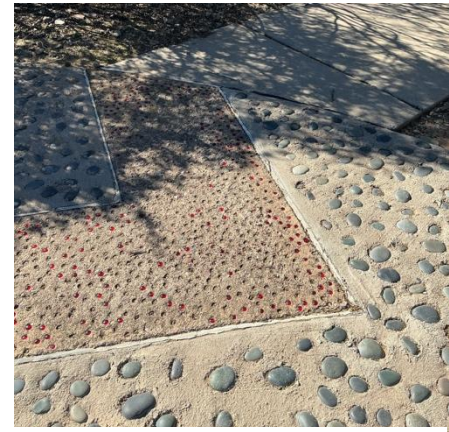
Uneven Path Surface
