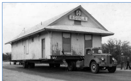
The Aguila train depot purchased for the McCormick-Stillman Railroad Park was moved from Aguila to Scottsdale in October 1977. Scottsdale Public Library photo
