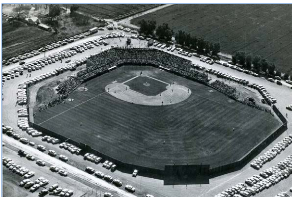
The Scottsdale Baseball Club raised funds in 1955 to build Scottsdale's Cactus League ballpark on Osborn Road. The Baltimore Orioles were the first to hold spring training here, 1956-58. After the Scottsdale Charros formed in 1961, they assumed spring training hosting duties from the Scottsdale Baseball Club, and have worked with the Boston Red Sox (1959-65), Chicago Cubs (1967-78), Oakland A's (1979-81) and the San Francisco Giants since 1982. Scottsdale Charros photo
