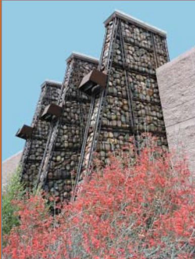
Artistic wall gabions help the Chaparral WTP blend into the surrounding landscape of the Scottsdale Xeriscape Garden.
