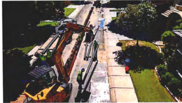
Gainey Village Casitas Waterline Replacement
