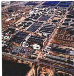
91st Avenue Wastewater Treatment Plant
