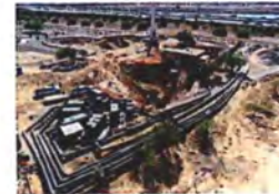
COS Princess Metering Station Rehabilitation
