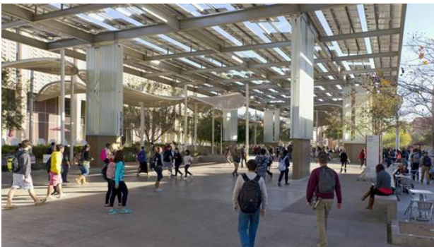
Pedestrian solar PV shade canopy.
