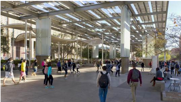
Pedestrian solar PV shade canopy.
