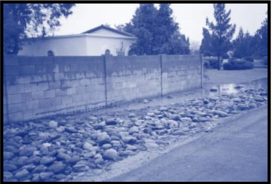
Undersized wall openings clogged easily, and caused the flooding in the photo on the cover.
