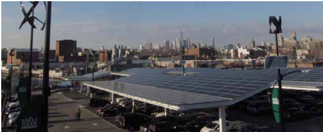
Rainwater capturing PV array at the Brooklyn Wholefoods
