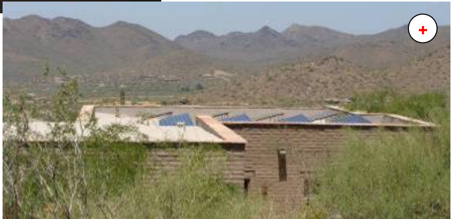
Solar panels on flat roof with parapets.
