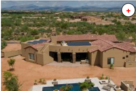
Solar panels on flat roof with parapets.
