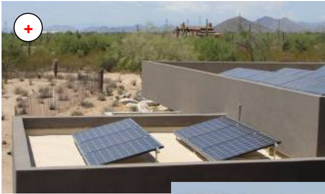
Solar panels on flat roof with parapets.
