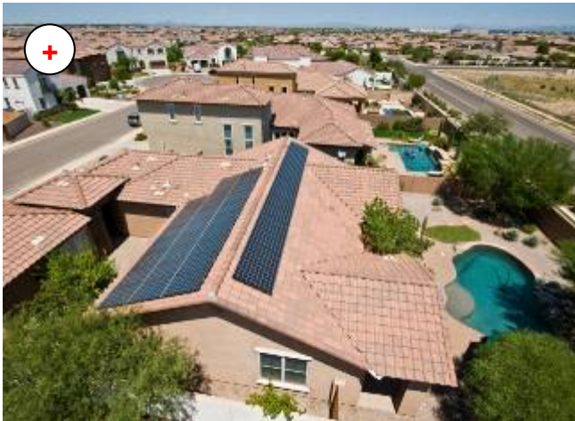
Solar panels on west and east facing pitched roof below the maximum allowable height of 24 inches above roof surface at any point.
