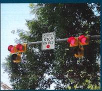
Example of PHBs mounted on a mast arm. Source: FHWA
