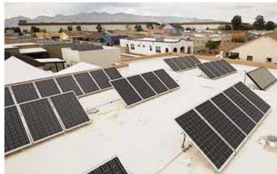
Homebuilder John Wesley Miller's "net zero energy" all-electric homes feature photovoltaic panels that provide as much energy as the home uses.
