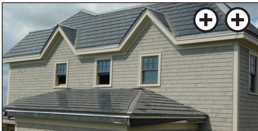
(Illustration 23) Photovoltaic shingles are best integrated when they cover the entire roof so as not to contrast with the other shingles. Source: Atlantis Energy Systems.
