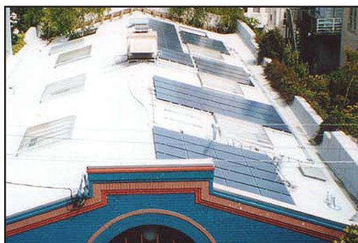
(Illustration 48) This commercial solar panel system on the San Francisco “Rosebud Agency building” is mounted flush with the roof behind a parapet system.
