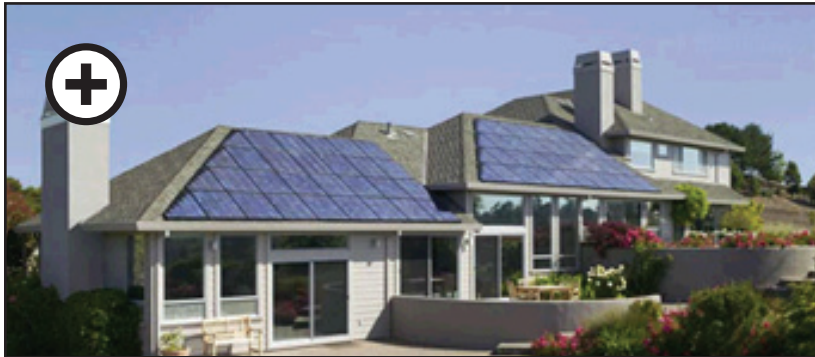
(Illustration 33) Triangular solar panels match the triangular roof planes on this home. Source: SPG Solar
