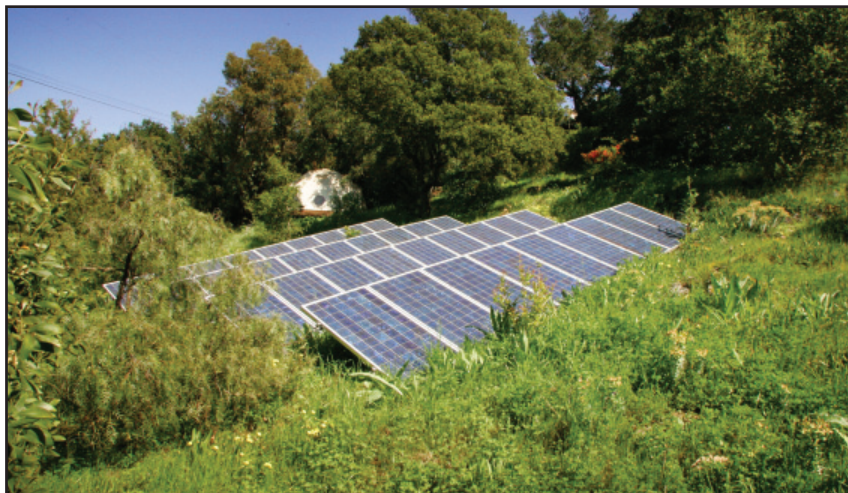
(Illustration 4) This photovoltaic array produces electricity that is used to power a nearby home.
