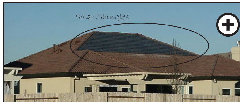
(Illustration 21.) Category 1: An example of building integrated solar energy system technology. Source: Atlantis Energy Systems.
