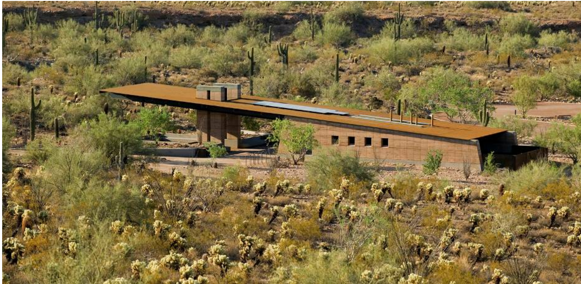
Lost Dog Wash Trailhead Building - McDowell Sonoran Preserve
