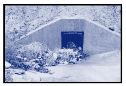
Trash and debris clog the drainage system reducing the flow of water and polluting our parks, streams, and lakes.
