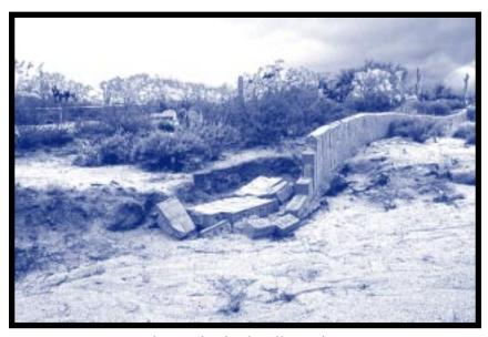
Inadequately sized wall opening.
