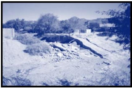
Severe erosion in an improperly lined channel.
