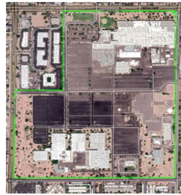
8201 E McDowell Road Building+asphalt fraction: 68.0% Building+asphalt area: 85.9 acres Industrial (3099)
