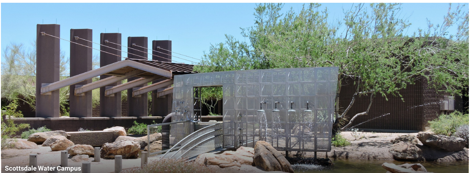
Scottsdale Water Treatment Plant
