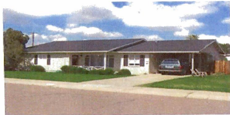
Original carports were for either one or two cars and were located on one end of the front façade under the main roof. Roofs were typically gable, like the one above, or hip roofs.
