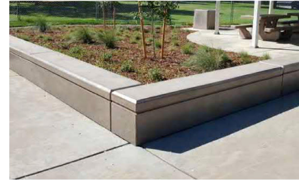
Cast-In-Place Seat Wall
