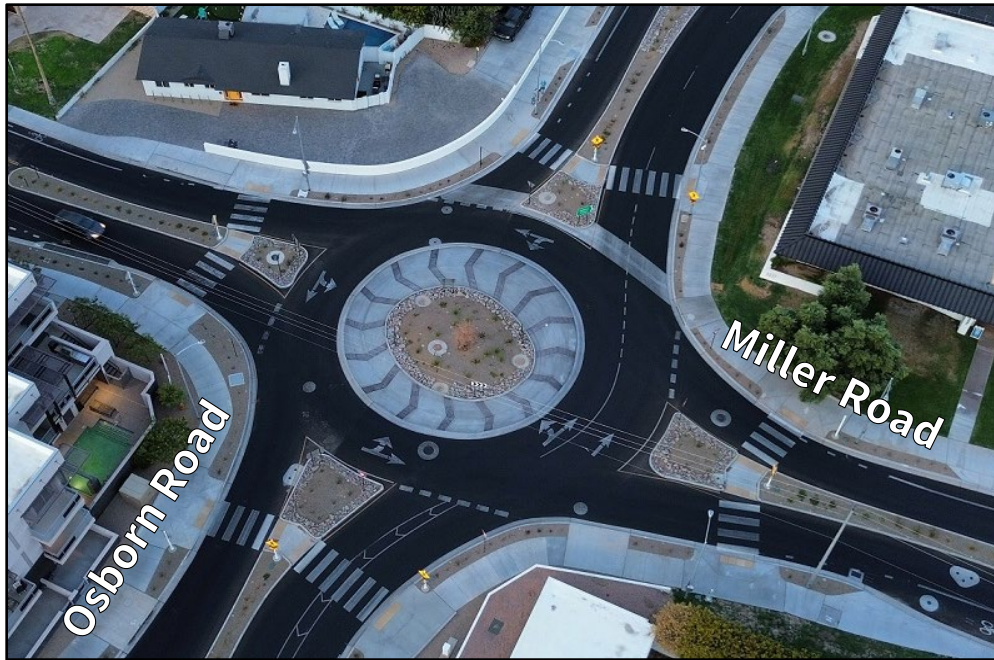
Figure 20: Aerial View of Miller Road and Osborn Road (2023)
