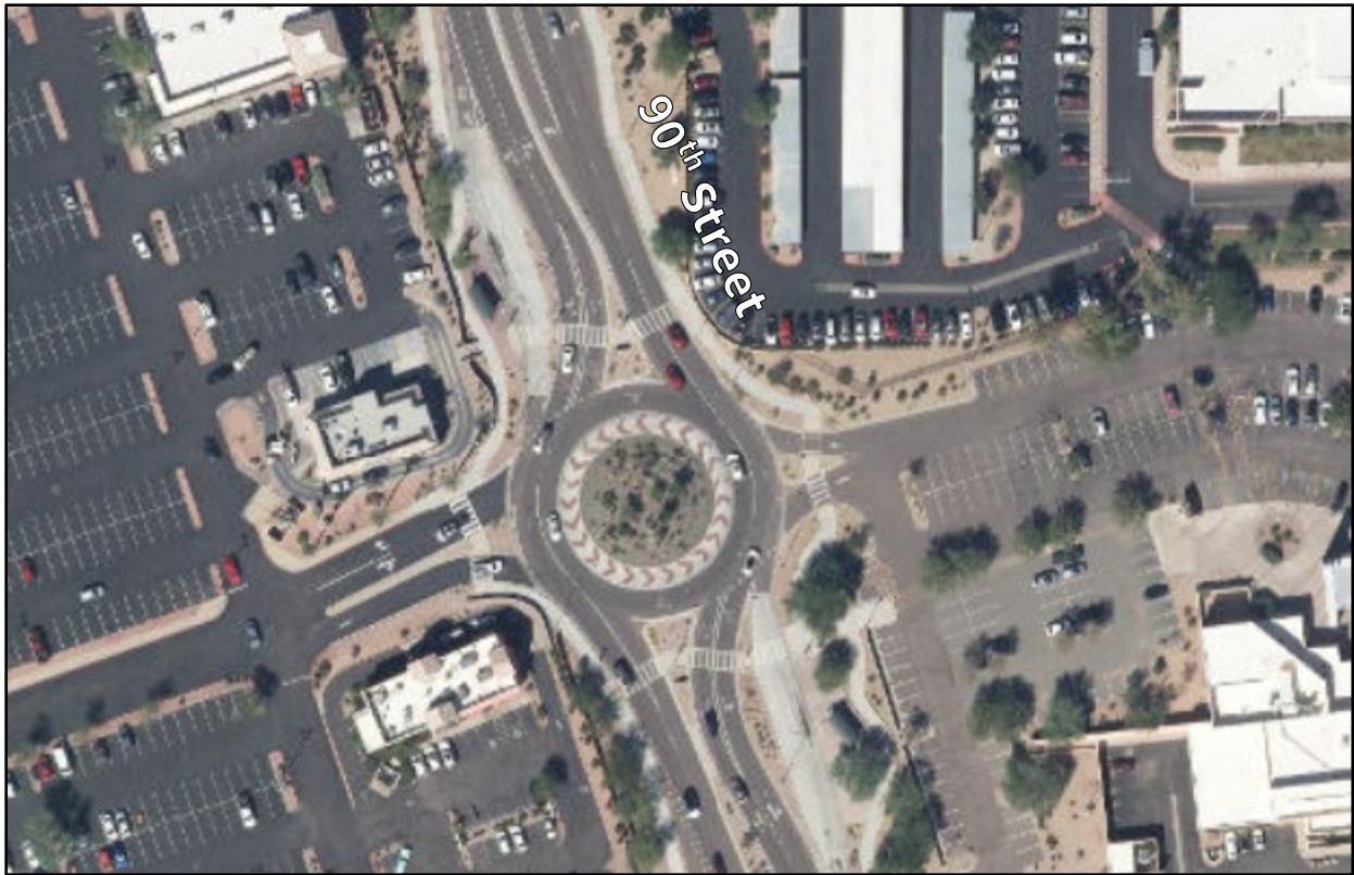
Figure 12: Aerial View of 90 th Street at Mustang Library Roundabout (2022)
