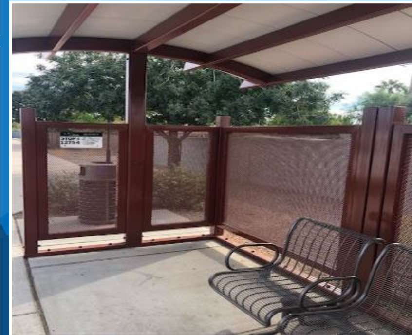
Refreshed with Electrostatic Red Oxide
