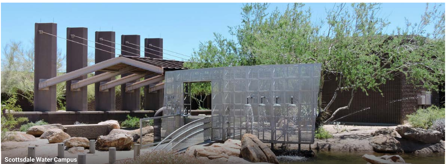
Scottsdale Water Treatment Plant
