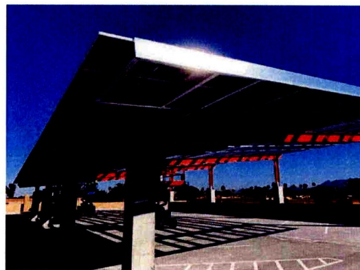
View of shade structure
