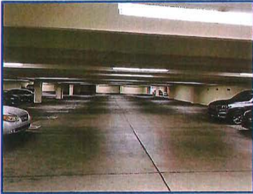
Brown Street Garage
