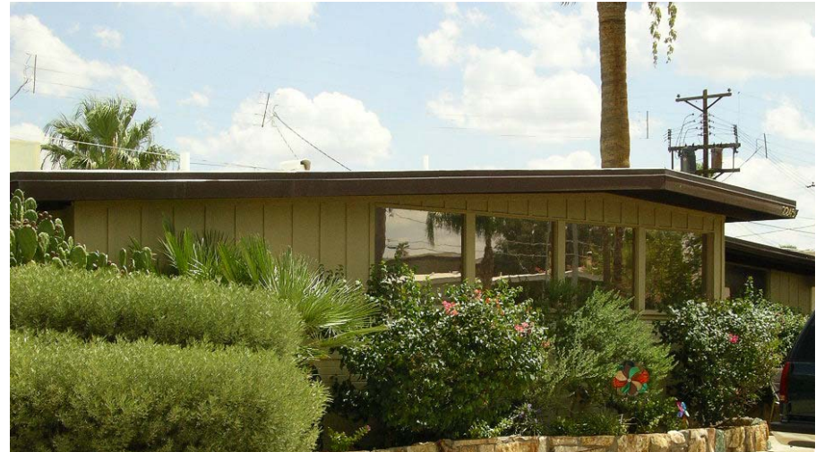
The board and batten siding and window-band are original elements. Use of wood on the upper half of the house was comparatively rare. All examples of wood siding are therefore important to retain.
