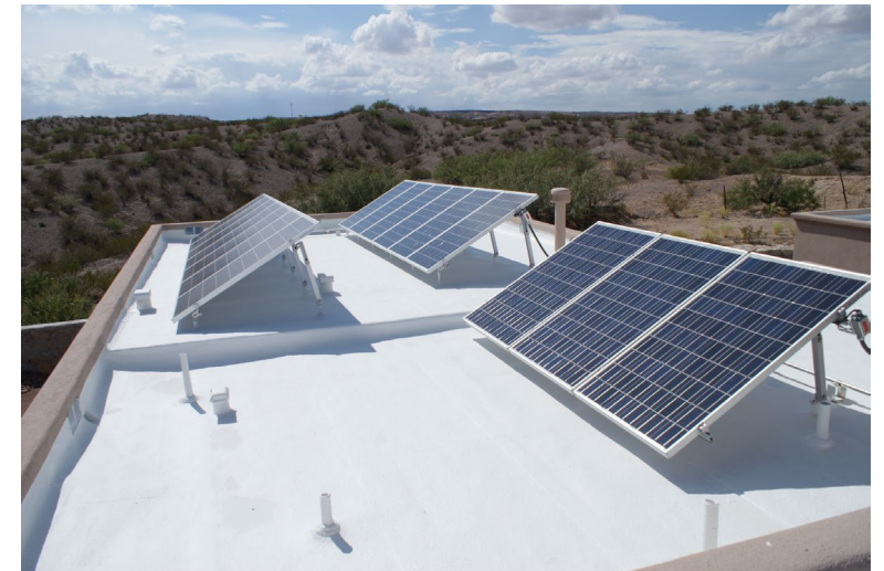
Credit: Carlisle Roof Foam
