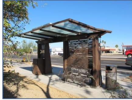
Shade structure and amenities
