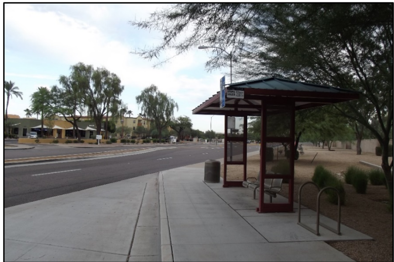
Scottsdale standard bus shelter and associated amenities
