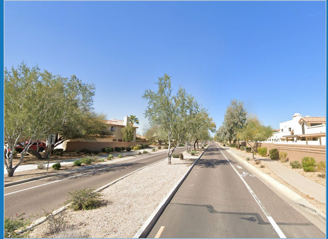
Minor Collector 96 th Street - After
