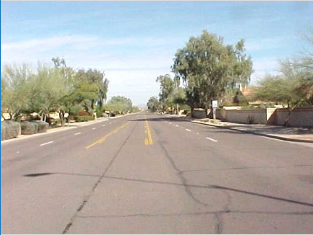
Major Collector 96 th Street - Before
