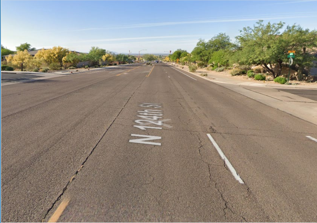
Major Collector 124 th Street - Before
