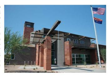
The contemporary architecture responds to both the civic & historical context of the surrounding urban area drawing from the materials, colors, and textures of the existing built environment. Natural materials including locally manufactured ground face concrete masonry, in combination with Arizona sandstone, glass, and weathering steel define the building surface and exude a sense of sustainability and presence.
