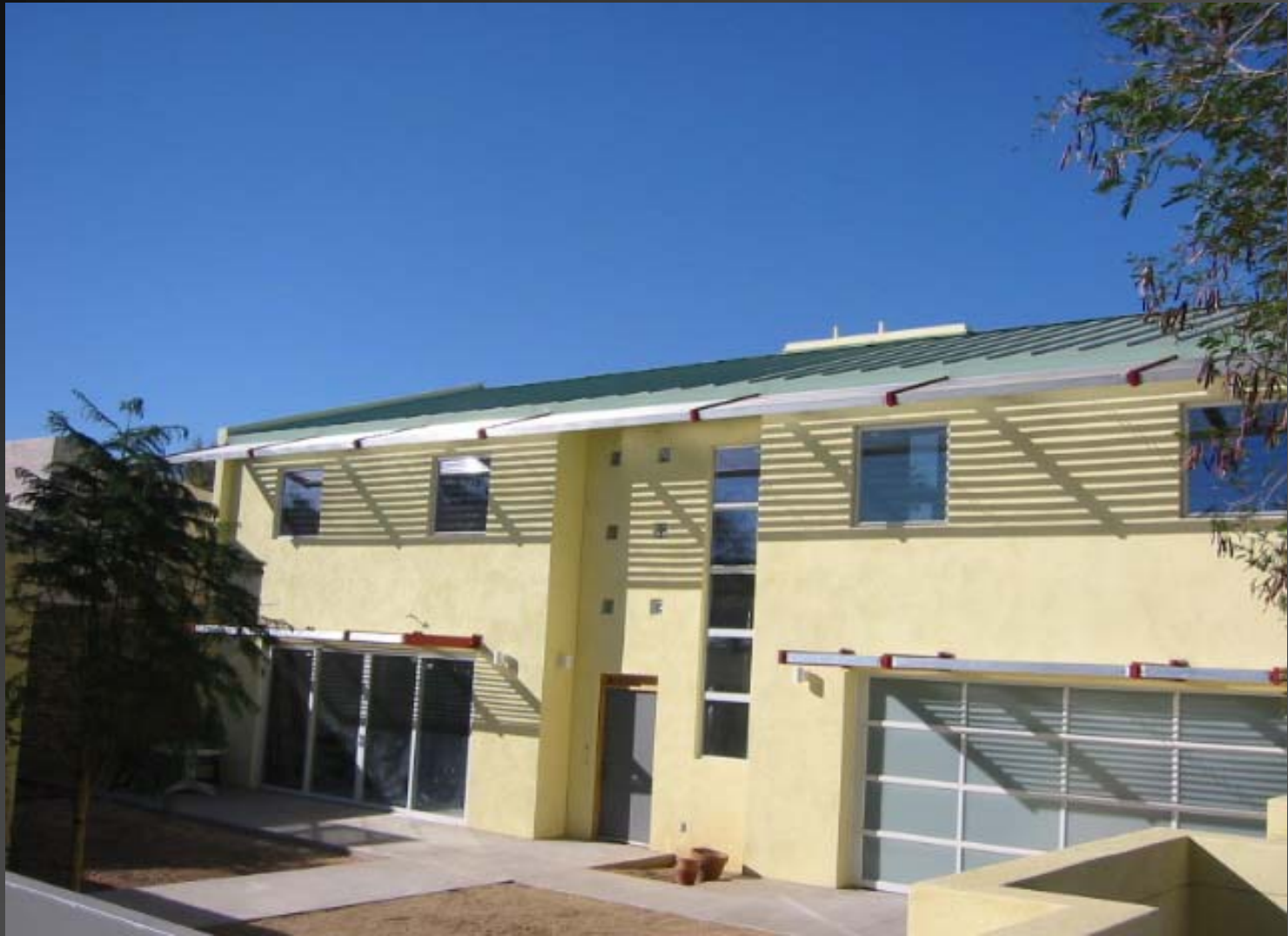
Louvered Overhangs - South Elevation on October 18 McDonnell House
