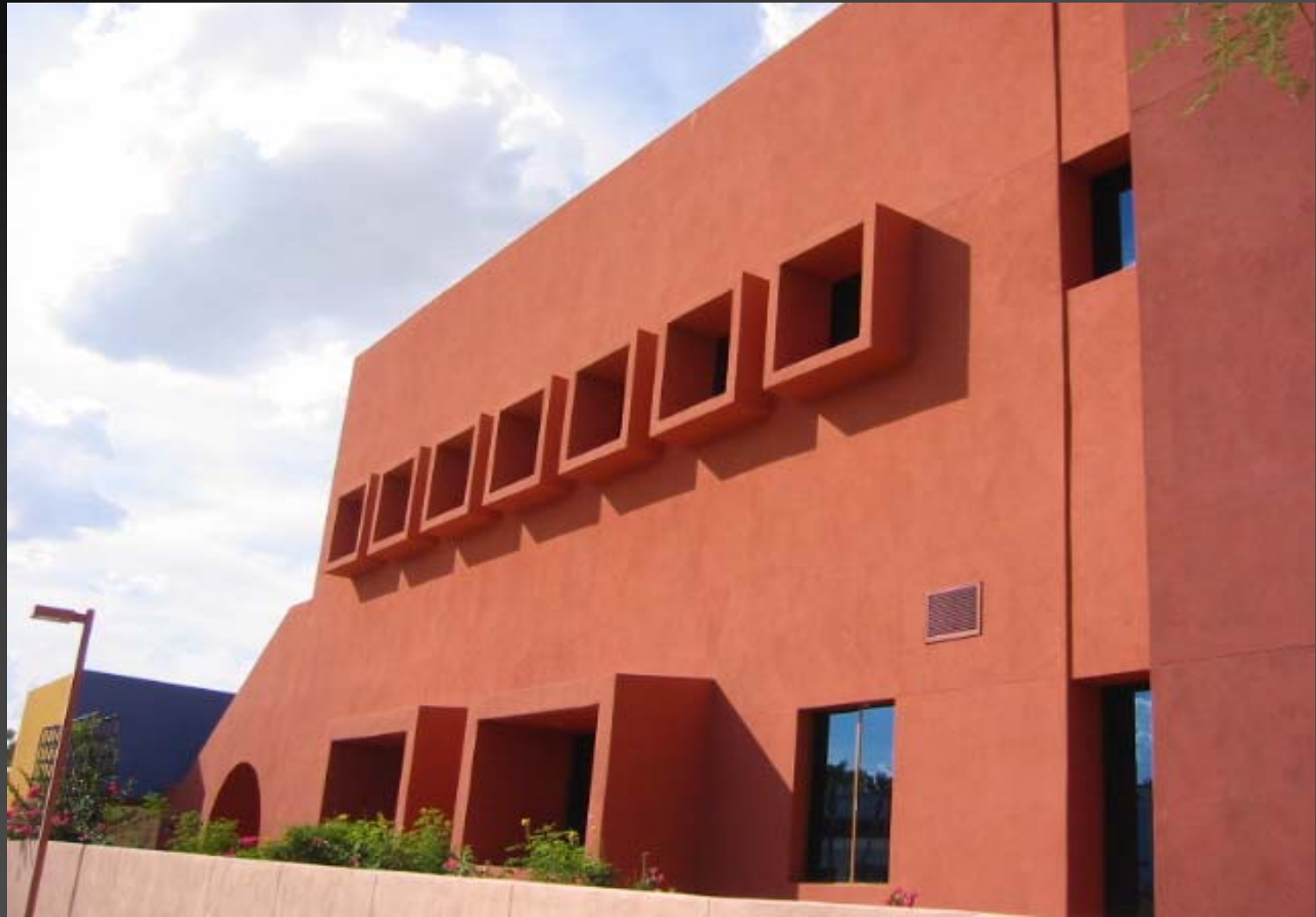
South Elevation in August
