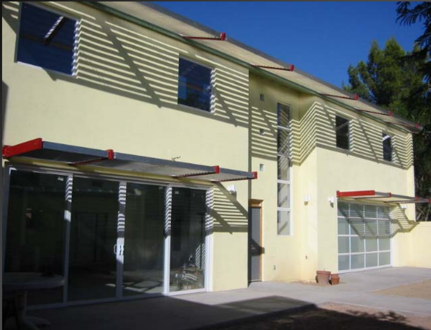
Louvered Overhangs - South Elevation on October 18 McDonnell House
