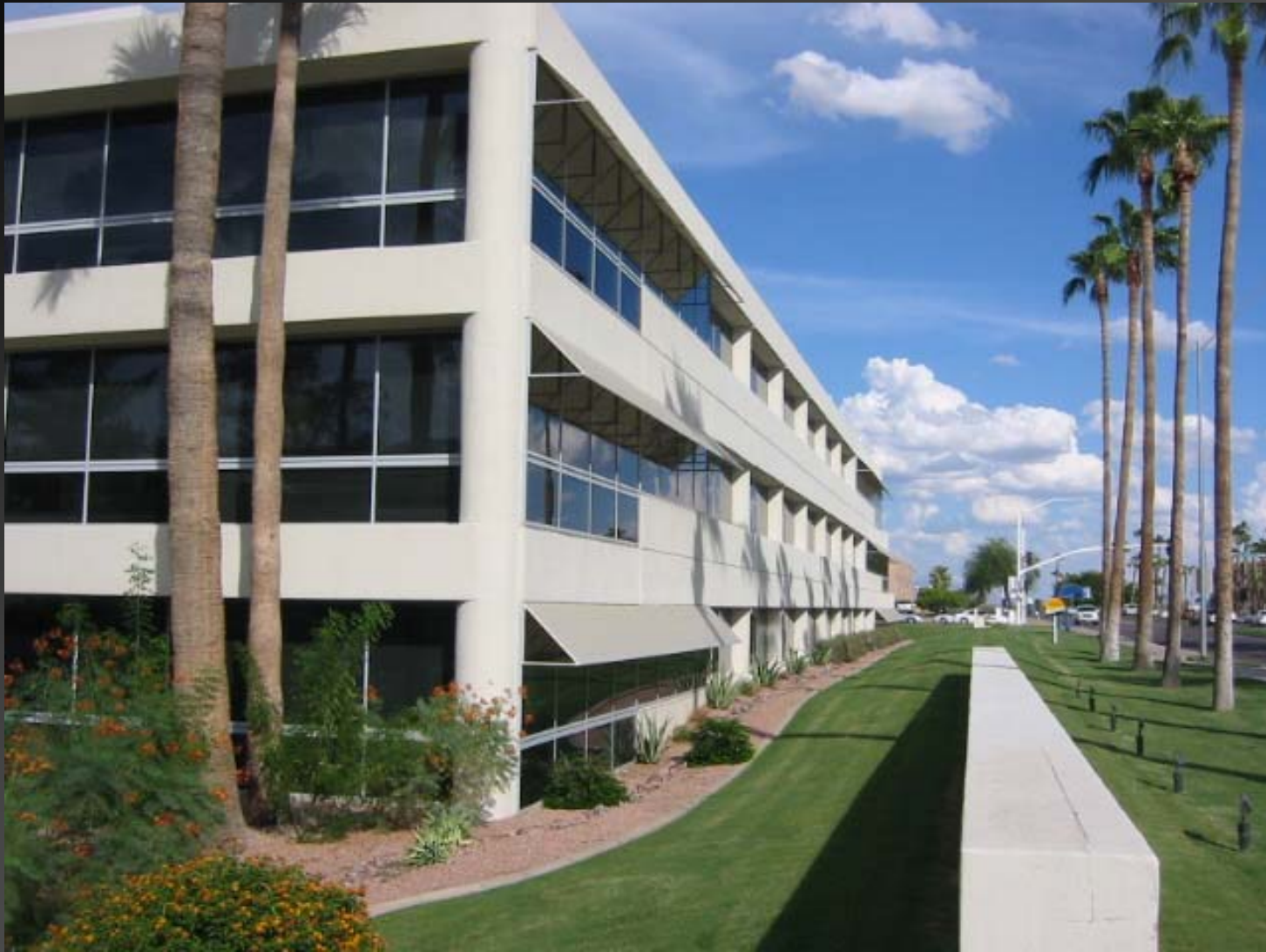
South Elevation in August
