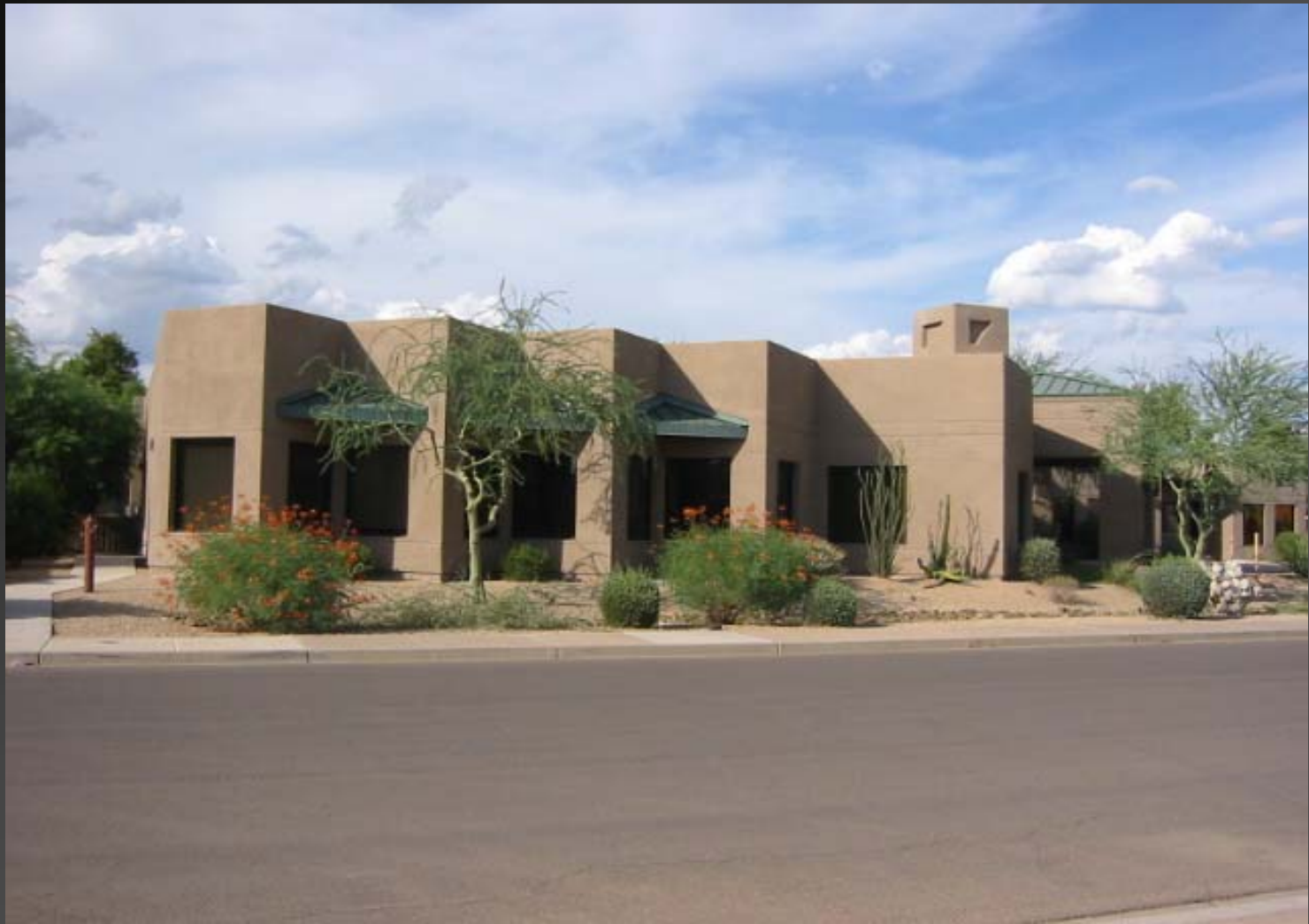
South Elevation in August
