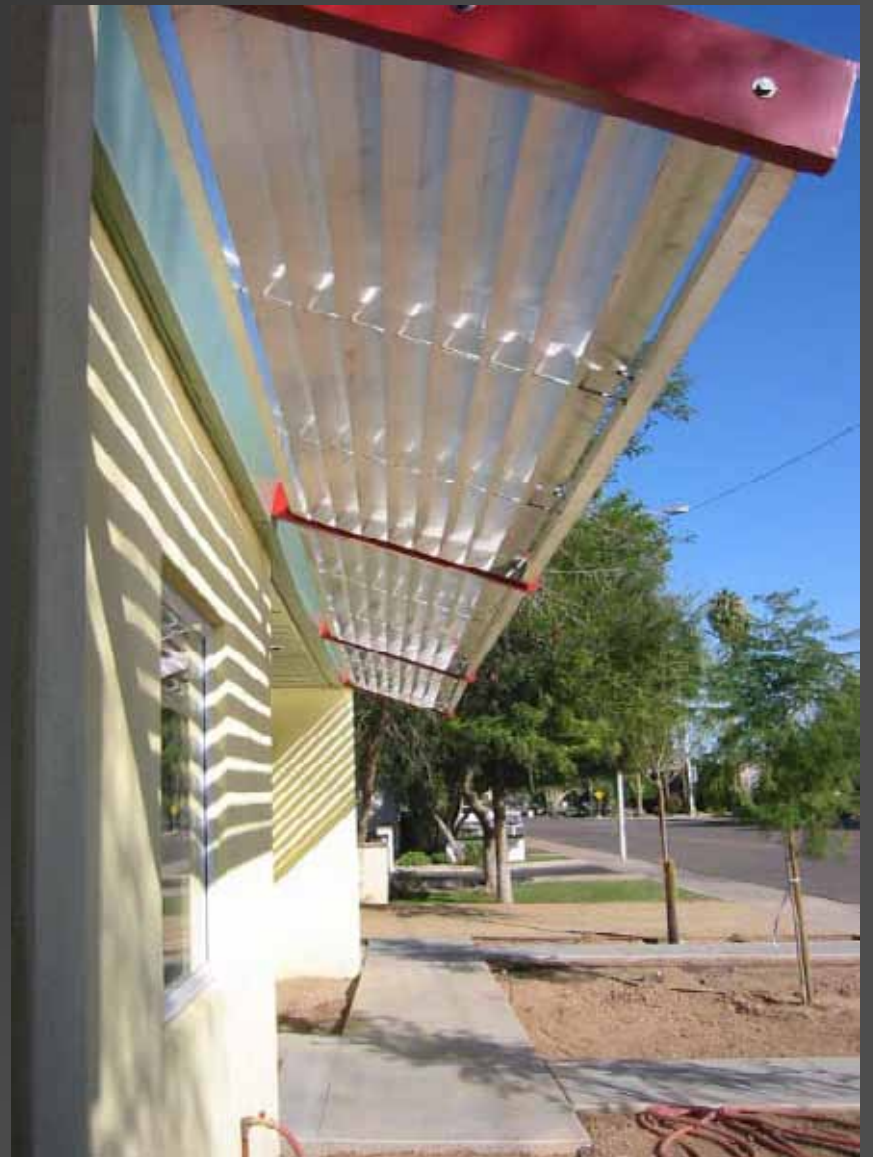
Louvered Overhangs - South Elevation on October 18 McDonnell House
