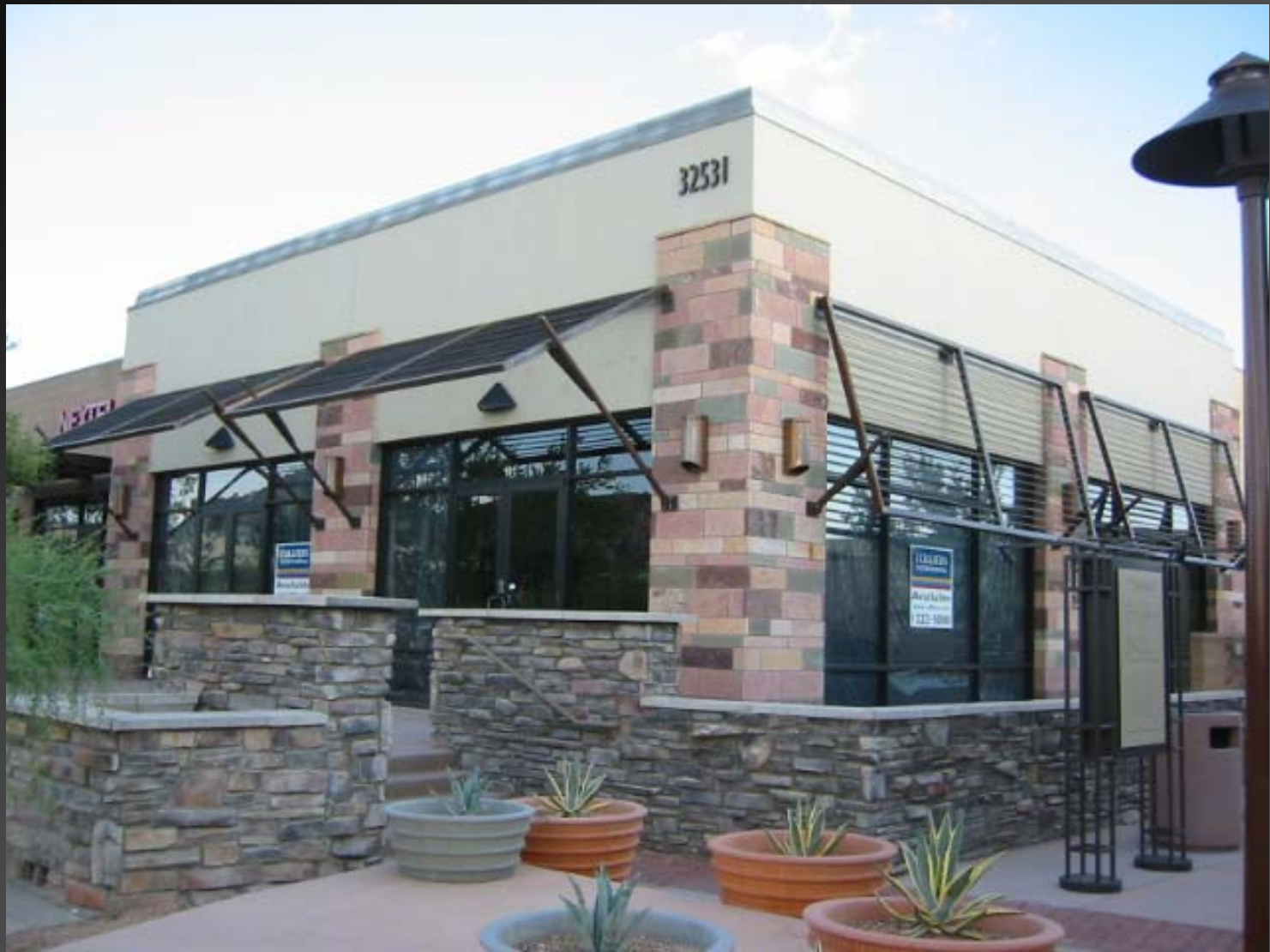
Southwest corner with fixed louvers Scottsdale Shopping Center
