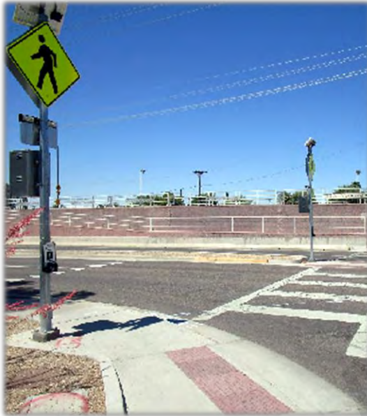
Rectangular Rapid Flashing Beacon
