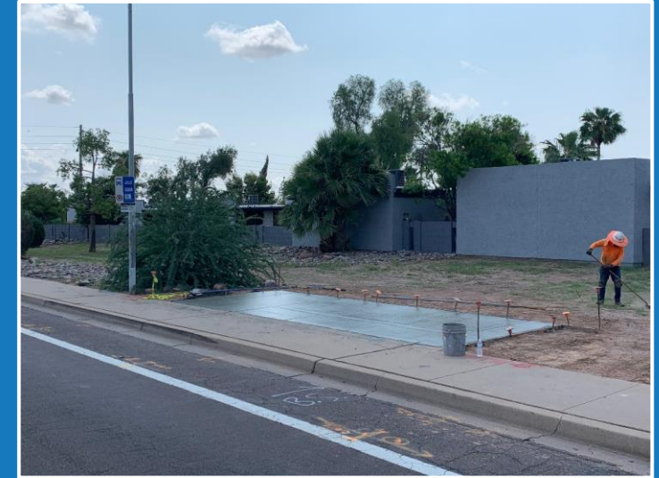
Pouring of new bus pads
