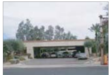
Driveways along the pedestrian route limits continuity (photo taken in Downtown).
