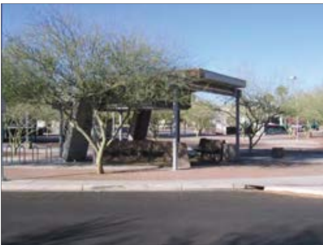
An example of a shade structure at Loloma Station
