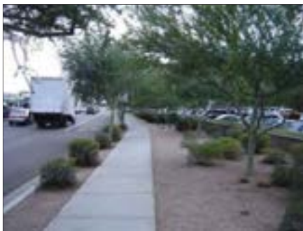
This separated sidewalk includes landscaping on both sides of the sidewalk to shade pedestrians and provide a physical separation from traffic (Scottsdale Road near Greenway-Hayden Loop).
