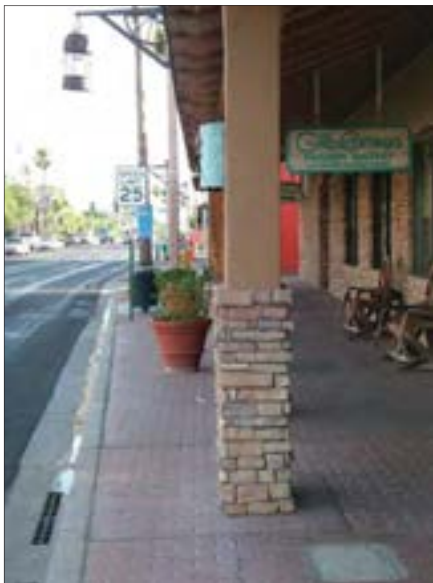
Narrow and cluttered sidewalks can impede pedestrian accessibility and mobility. Heavily textured paving with gaps greater than 1/4-inch can create uneven and bumpy surfaces (Scottsdale Road).
