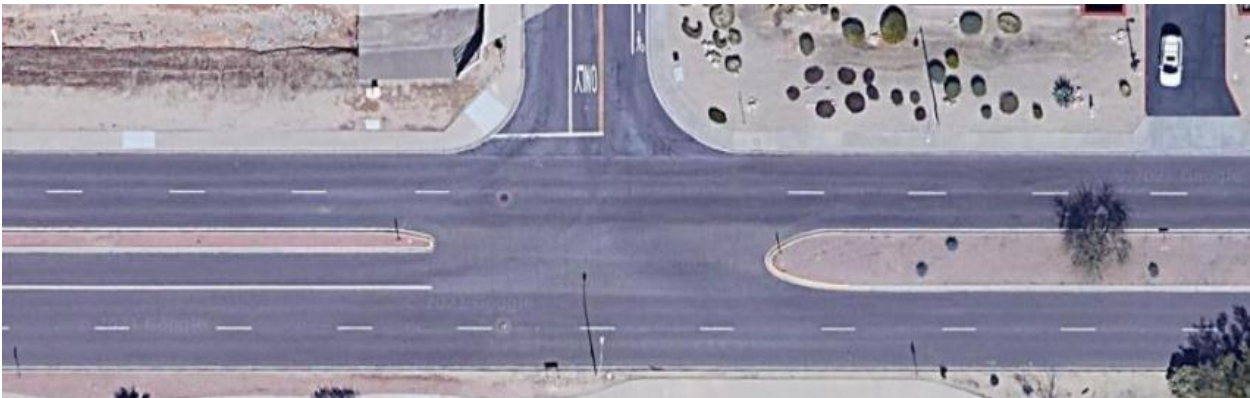
Figure 2.3: Aerial view of Via Linda and 108 th Street – Control Site (#28) (Google, 2021)
