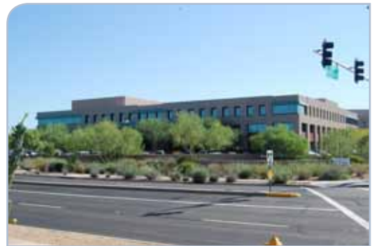
Henkel Headquarters (top) and Vanguard (bottom) are examples of business expansion and retention in the Greater Airpark. Photo source (top): Henkel
