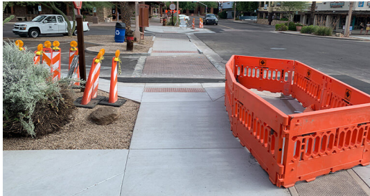
Newly installed ADA ramp in Old Town.
