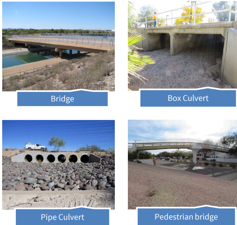
Figure 5. NBIS Bridge and Culvert Examples
