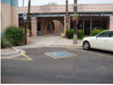
Main Street Arts – ADA parking with no ramp
