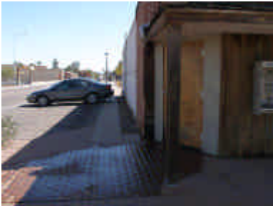
Old Town – lack of ADA walkway and ramps
