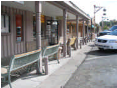
Old Town – boardwalk clearance issues
