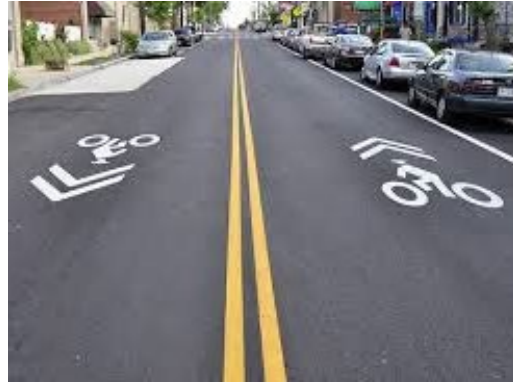
Asphalt Sharrow with on-street parking on both sides
