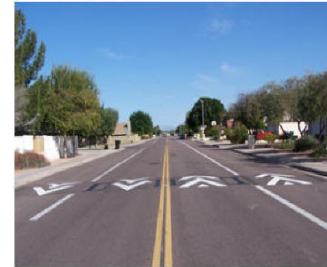
Traffic calming: speed cushion
