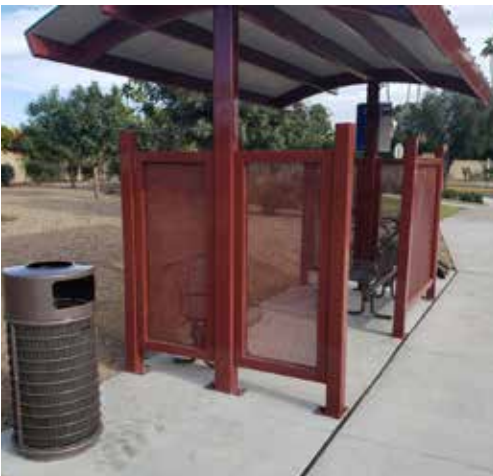
New bus shelter at Mountain View-Arbic
