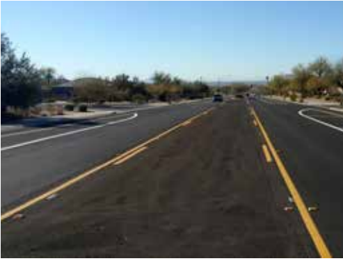
New pavement and striping on 124th Street
