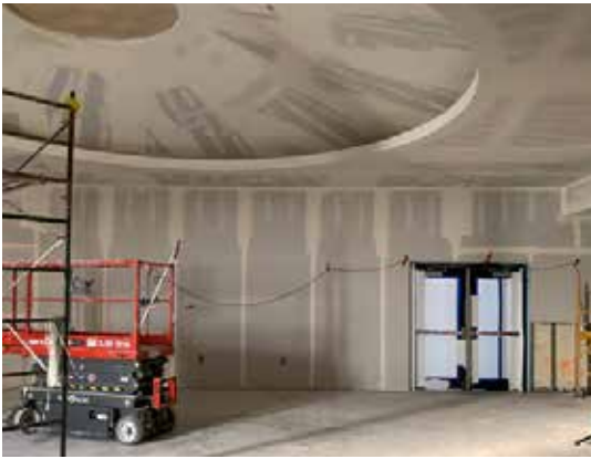
Civic Center storytime room construction
