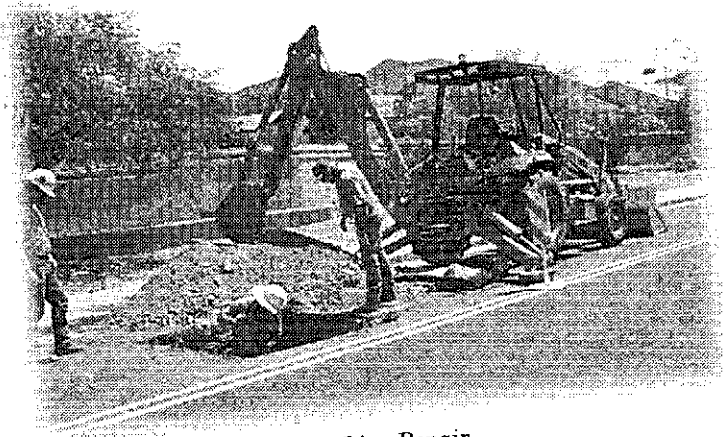
Water Service Line Repair
