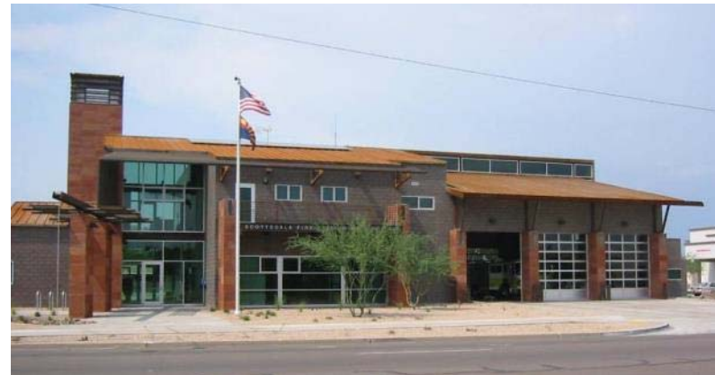
Downtown Fire Station 2 - Platinum
