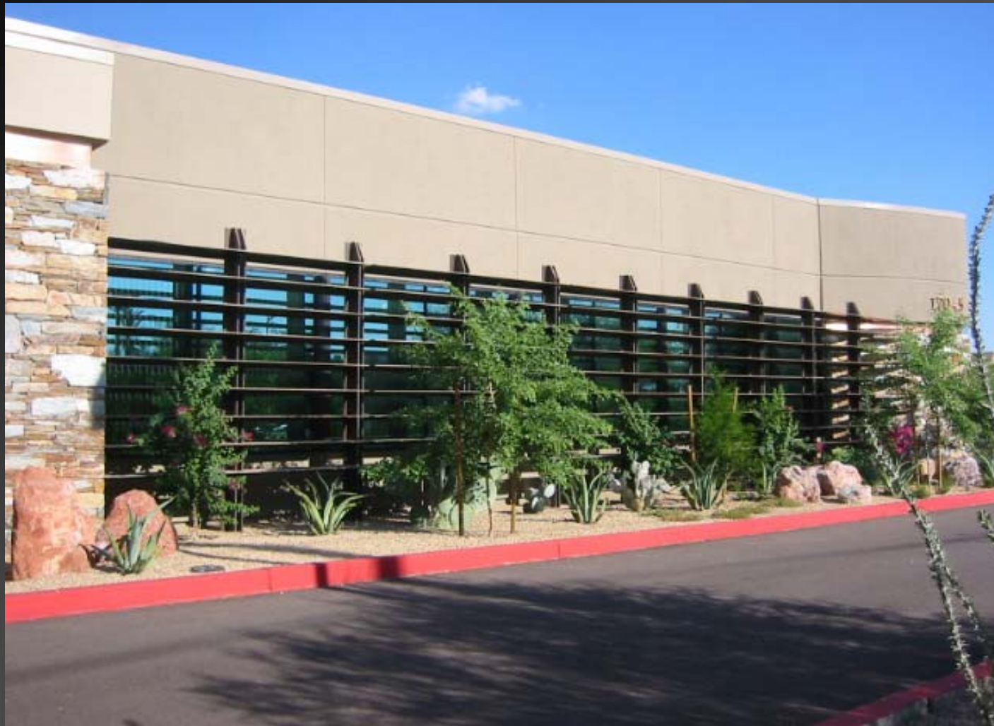
Louvers (mini-overhangs) on West Elevation in August
