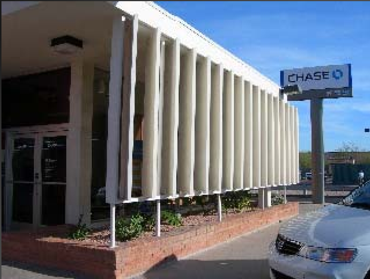
West Elevation at Bank One Phoenix
