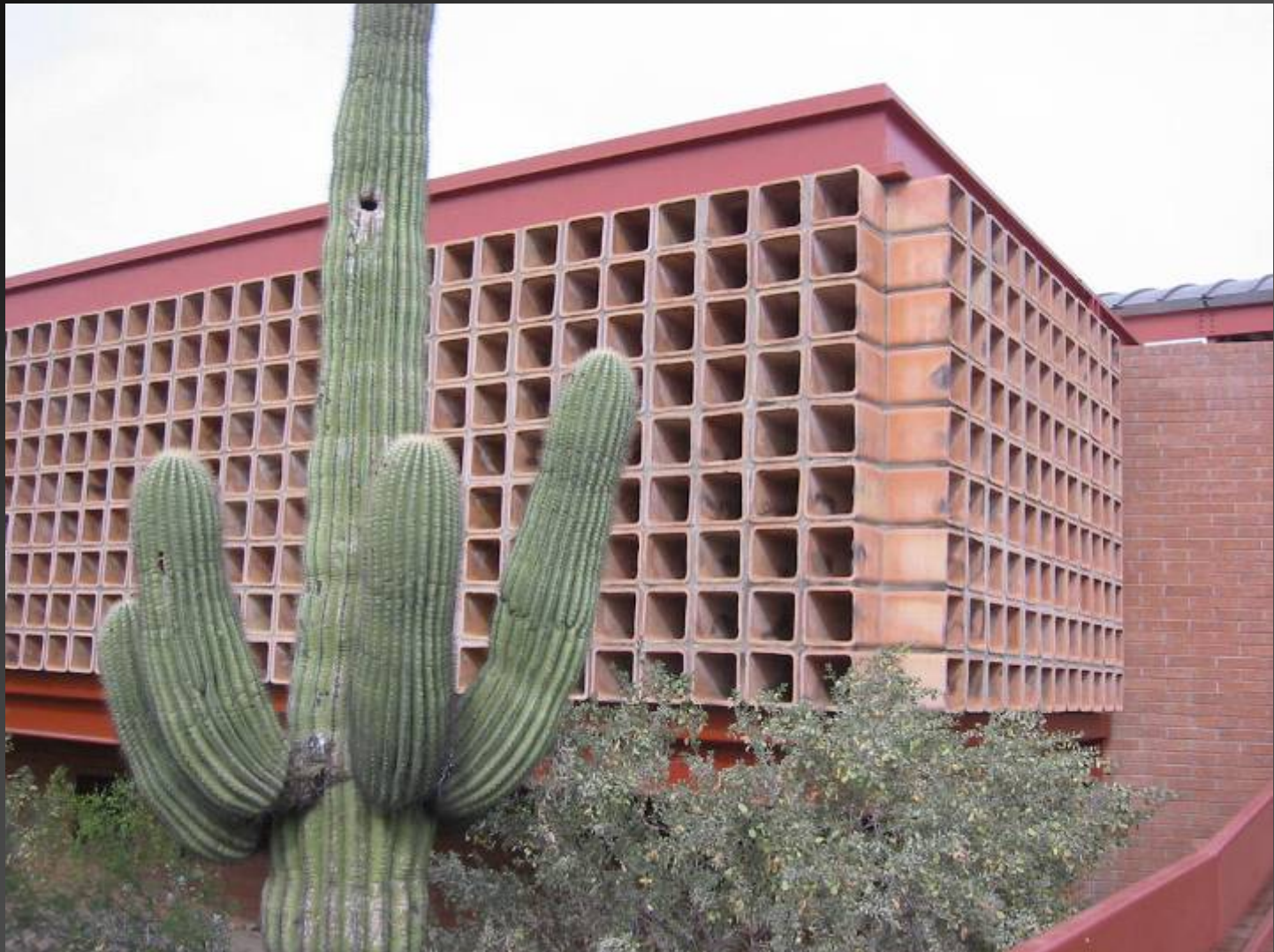
Chimney flue tile (16 x 16 x 24) wall on west facade AZ Cardinals Training Facility (Jones Studio, 1988)
