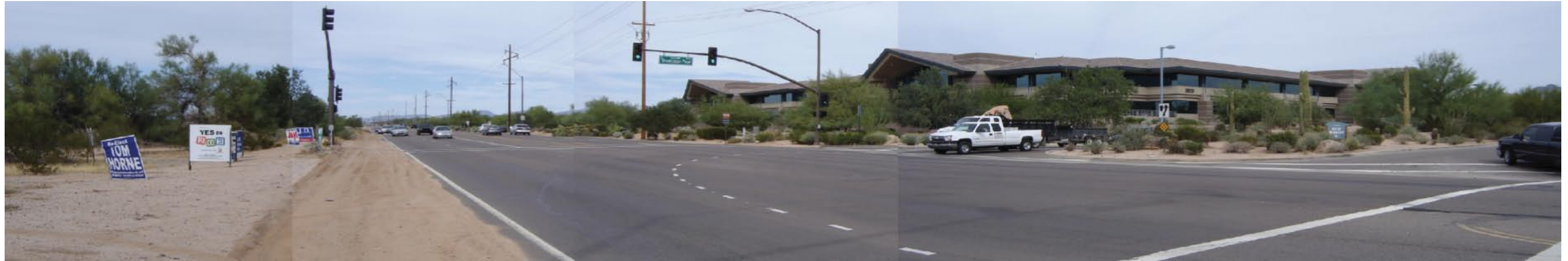
Existing conditions at Scottsdale Road and Thompson Peak Parkway intersection
