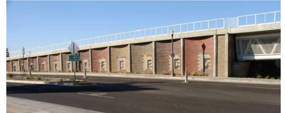
Buster Simpson's work with porcelain enamel panels and image inserts depicting a cracked Salt River mud motif on the south approach wall at Tempe Light Rail Bridge
