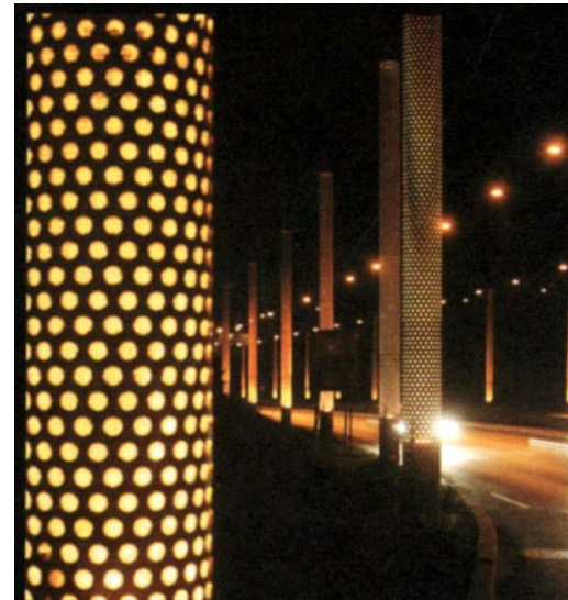
Light pole wraps to match decorative metal panels for the Segment I (Rivulet)
