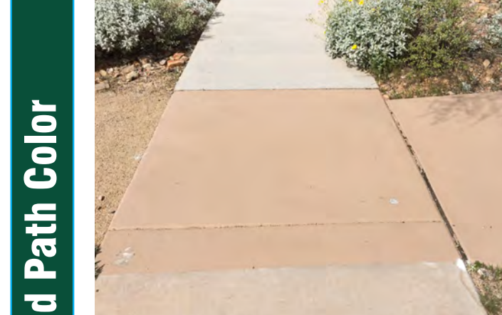
Proposed Path Color Integral Color “San Diego Buff” Multi-Use Path & Trail Connections
